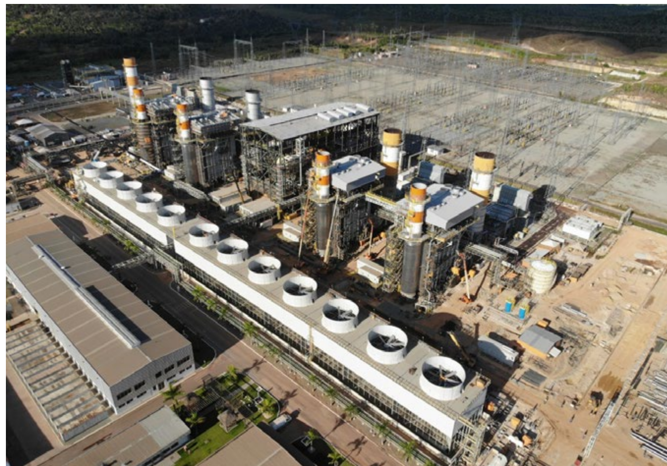
Parnaíba Complex and Transmission Line Substation in Santo Antônio dos Lopes, MA
