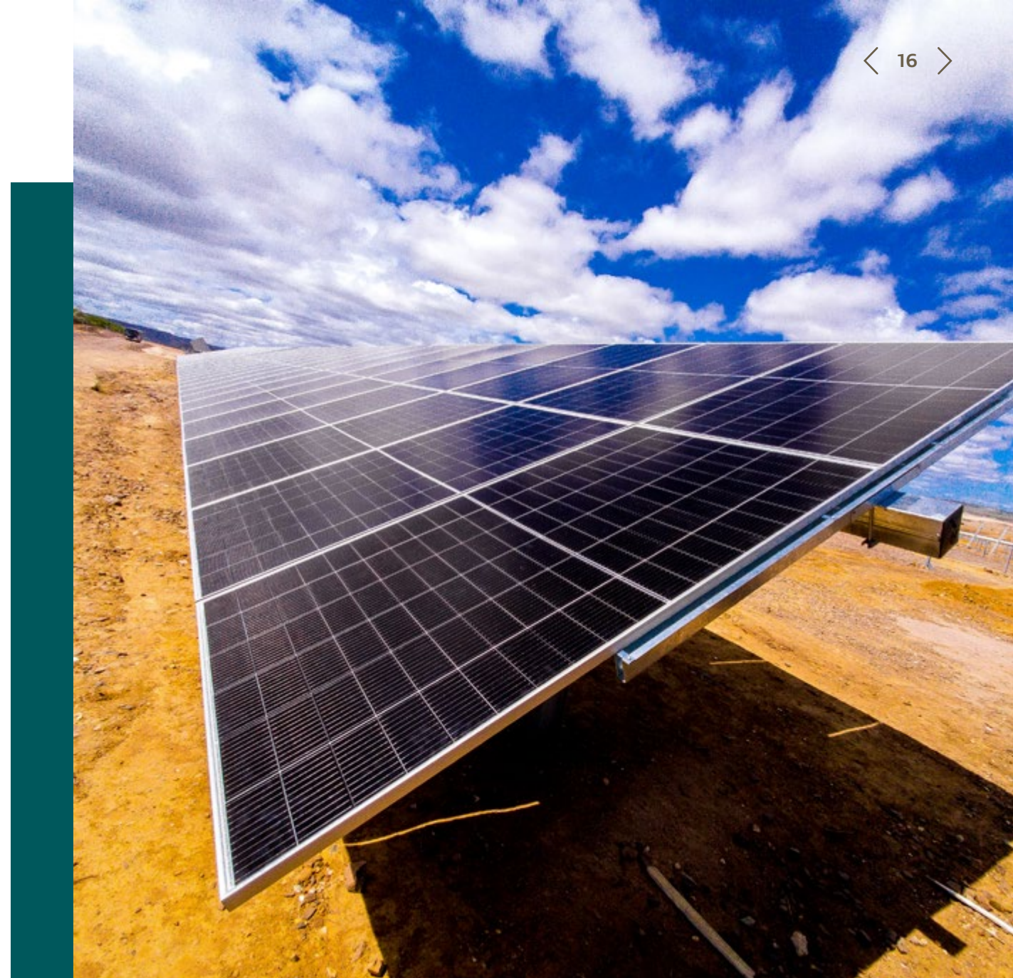
Futura I construction, Juazeiro, BA
