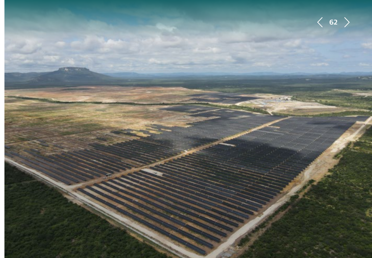
Construction of Futura I photovoltaic plant with 670 MW. Juazeiro, BA
