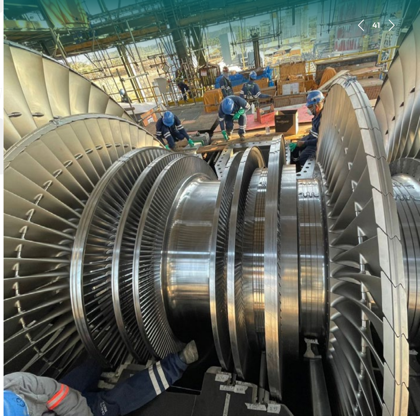
Steam turbine, Parnaíba V
